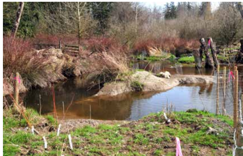
This small wetland was built in a low corner of a pasture within the riparian area of a creek in Langley.
